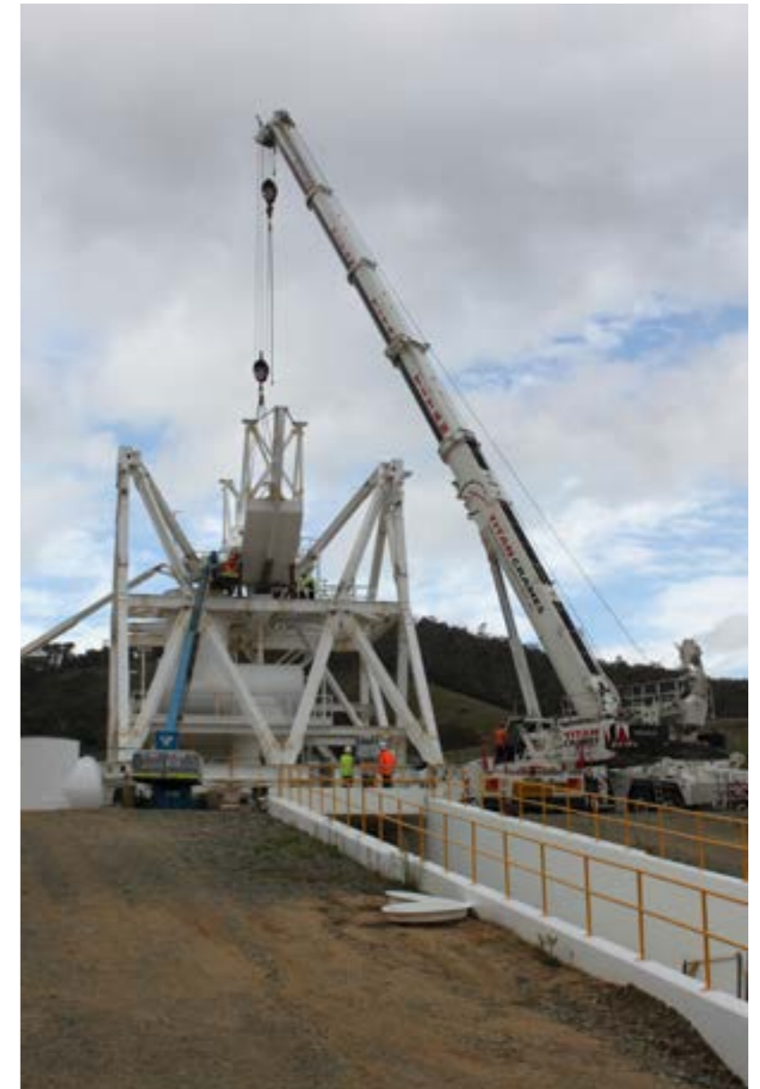
The second biggest crane lift of the project
